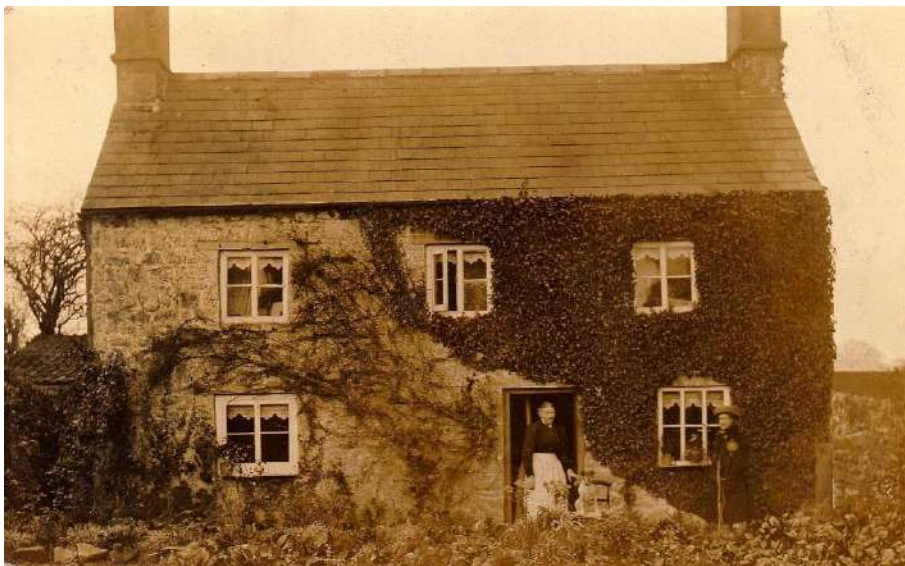
Ann's Cottage, Turner's Court Lane
